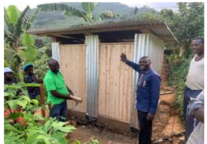
The newly constructed toilet at Kinyarushengye
